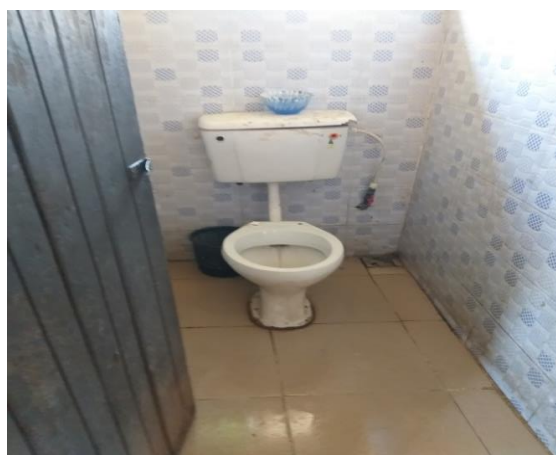
Plate 1D: A toilet facility in Evbareke market spare parts market.
